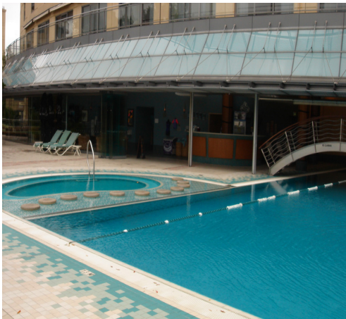
Star City's pool area after receiving the Sure-Grip treatment, exclusive to Non-Slip.
